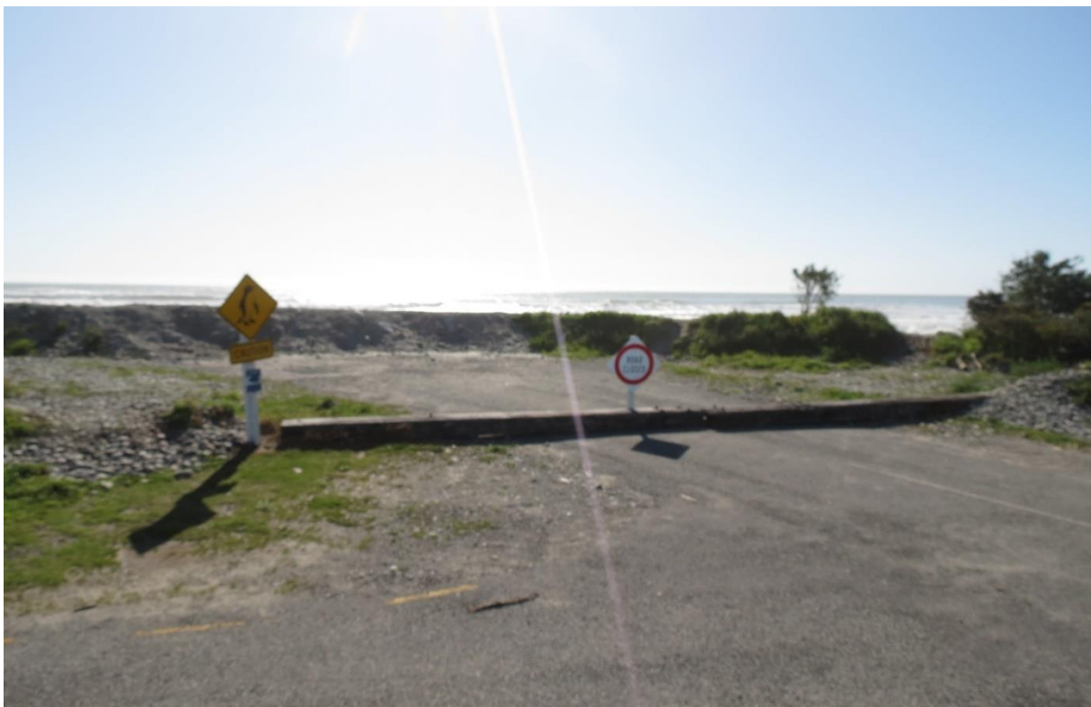
Figure A-6: Access to Hill Quay from Domett Esplanade, now closed to vehicles with a temporary gravel berm built on the former road surface. The roadway is a low-lying gap in the natural vegetated berm (just visible at right) and the buried 1969 revetment. [Credit: M. Allis (NIWA)].
