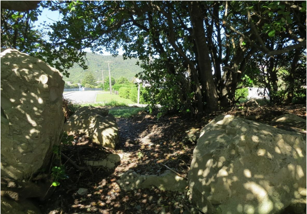
Figure A-4: Rocks from 1969 protection works within vegetated berm at Ward St. Date: 05-03-2020 [Credit: M. Allis (NIWA)].
