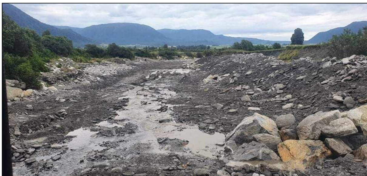
Photo shows section of Vine Creek that has been cleaned out
