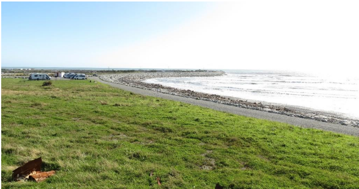
Figure A-2: View from former carpark along landfill and new revetment towards river mouth. Date: 05-03-2020 [Credit: M. Allis (NIWA)].
